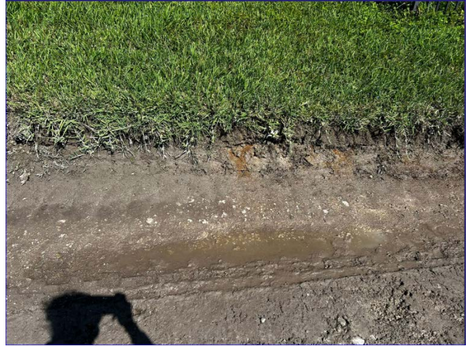
CLOSE UP OF THE ACCUMULATED WATER AND SEEPAGE
